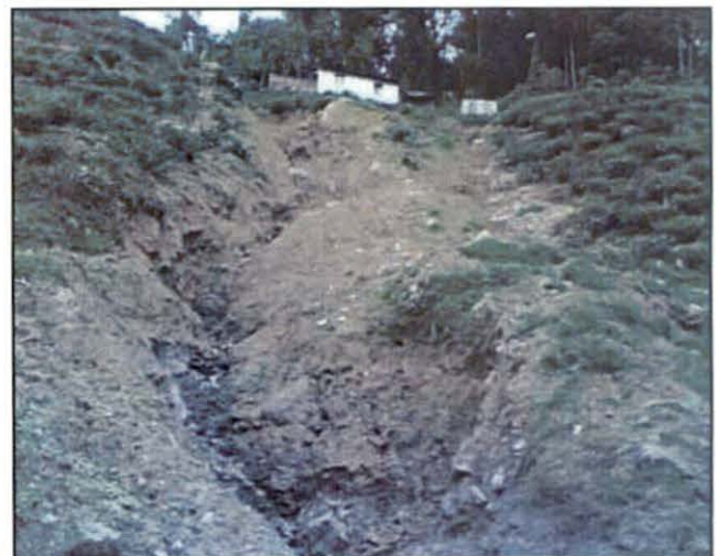
Photo 4.6 Slumping in Goomti Tea Garden, Kurseong
