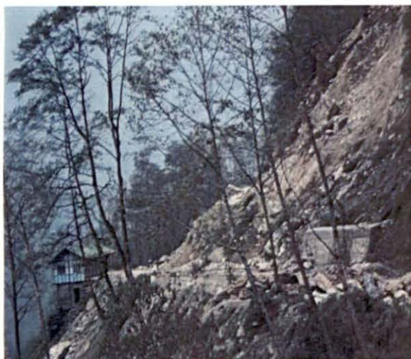
Photo 4.5. Debris slides near Kurseong
