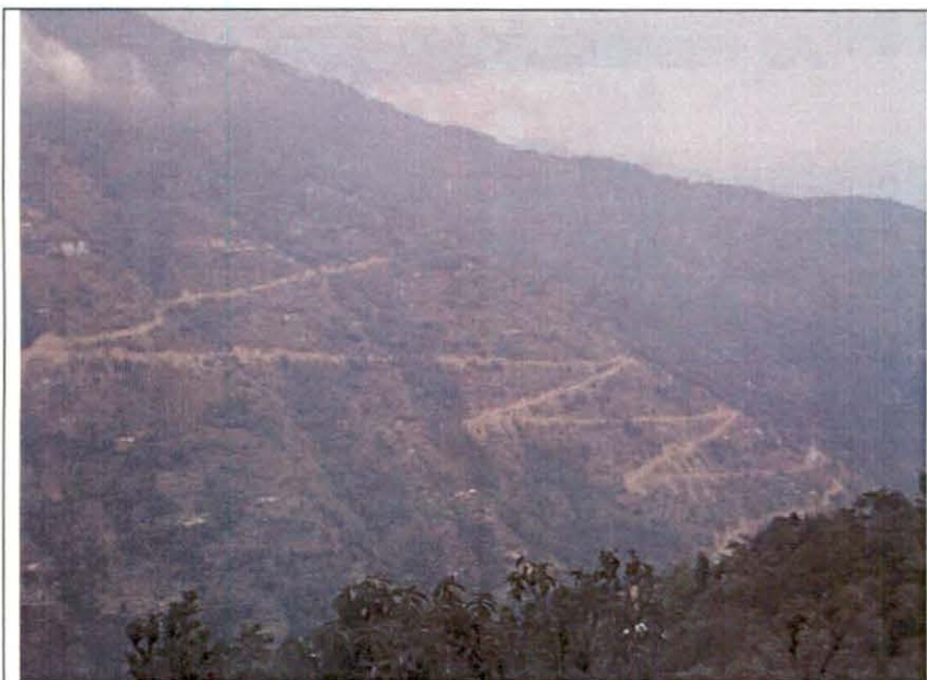
Photograph 8.3 Construction of motorable road near Rimbik caused innumerable landslides along the newly constructed road.
