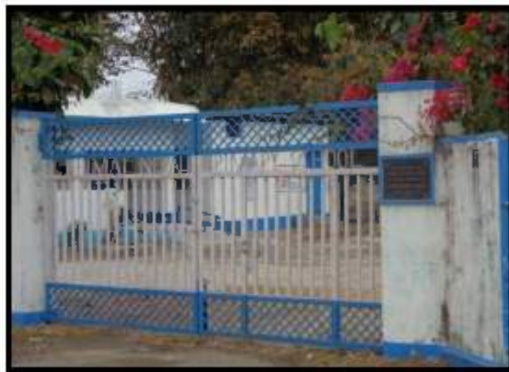
Plate 35. Primary School in Lower Bagdogra GP
