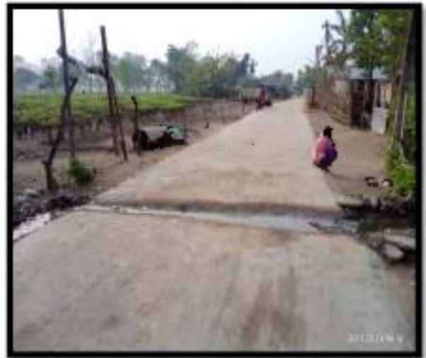
Plate 16. Drainage System in Tea Garden Area in Upper Bagdogra GP
