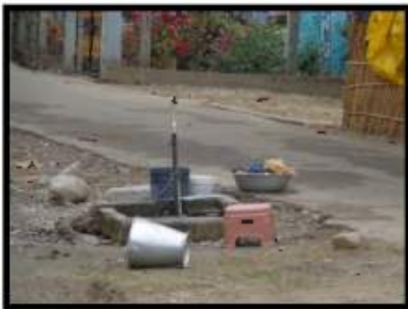
Plate 11. Drinking Water Facility in Lower Bagdogra GP
