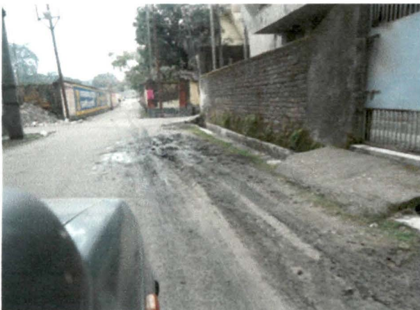
Drain Sludge on the Road Side
