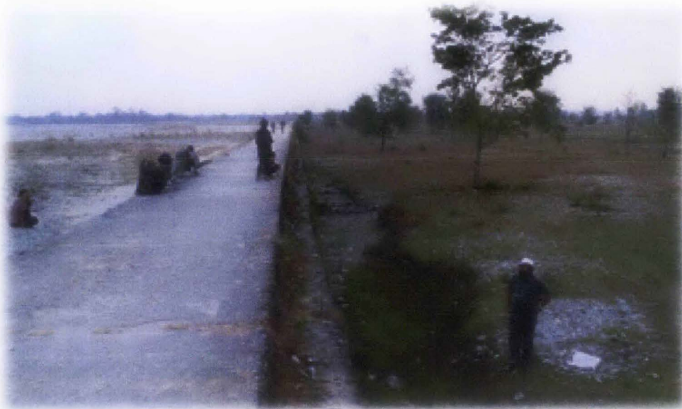
Photo 6.1. Embankment accelerates river deposition vis-a-vis rising of river bed at the Gish valley near Odlabari.
