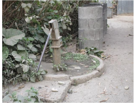
Plate 7.2: Dry Tube well, Gangaram TG
