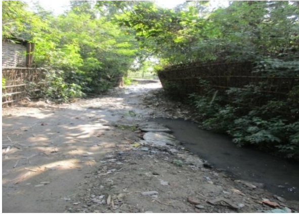
Plate 7.1: Poor road network, Shikarpur TG
