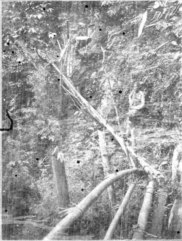
BRIDGE AT BEI, NEAR YANGYANG.
