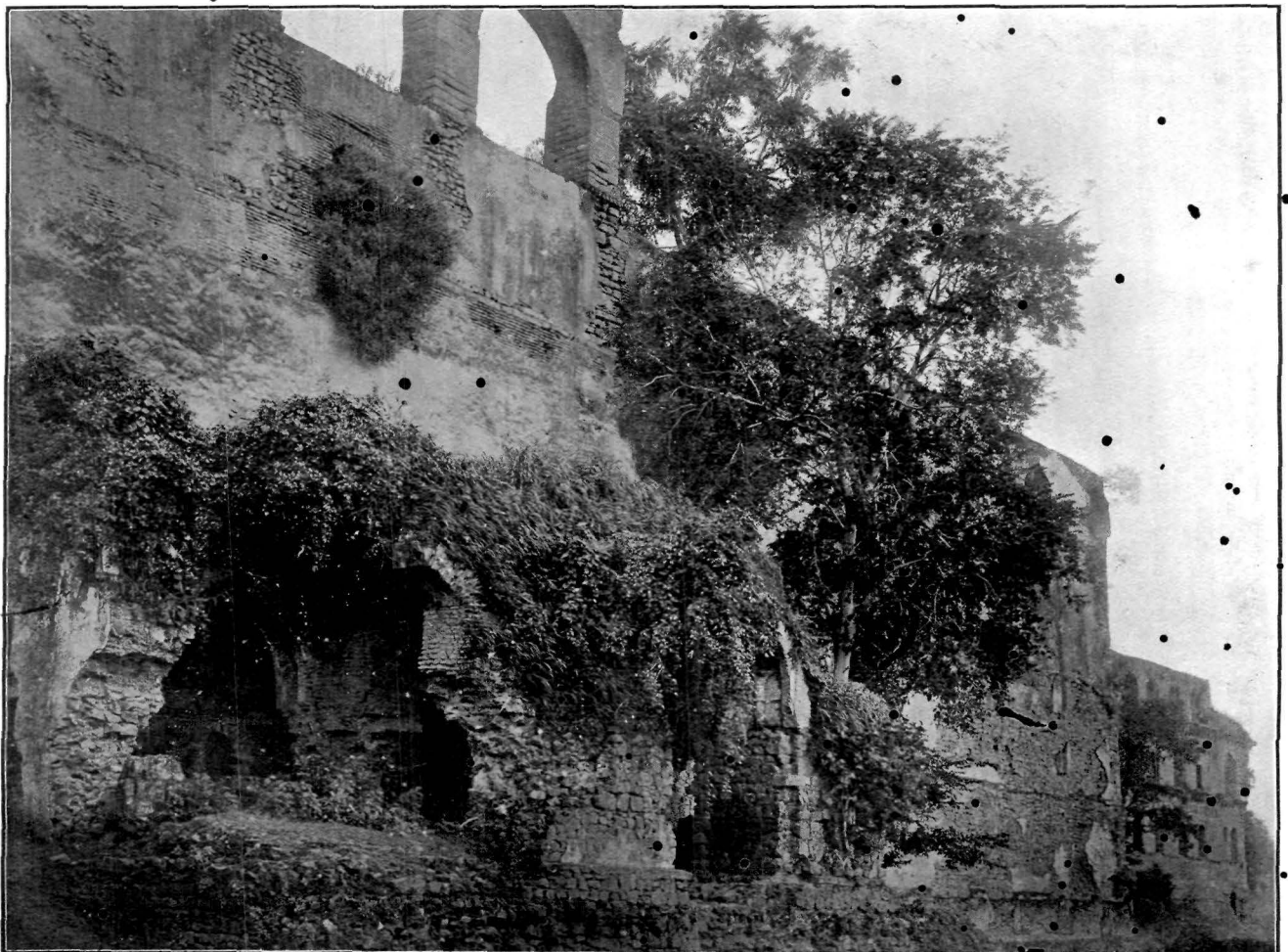
b. NEARER VIEW OF PALACE INSIDE THE FORT AT BURHANPUR, DISTRICT NIMAR.
