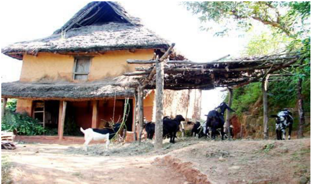
Figure: 10. Tamang House (surveyed by researcher in Nepal)
