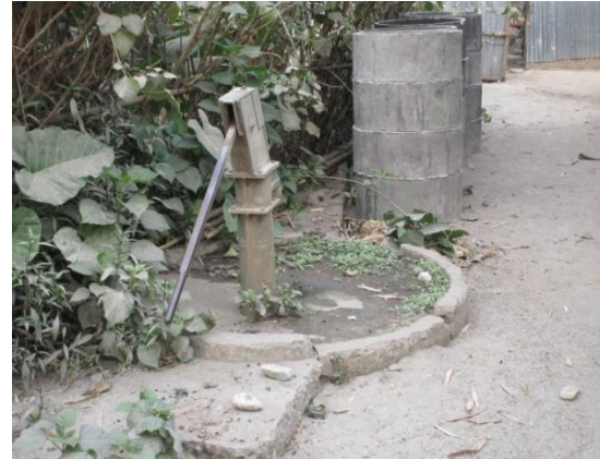
Plate 7.2: Dry Tube well, Gangaram TG
