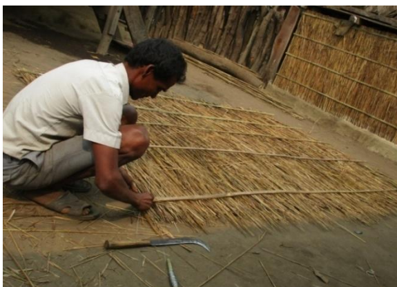
Plate 4.9: Houses repaired, Swaraswatipur TG
