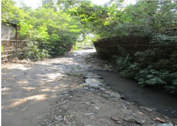
Plate 7.1: Poor road network, Shikarpur TG
