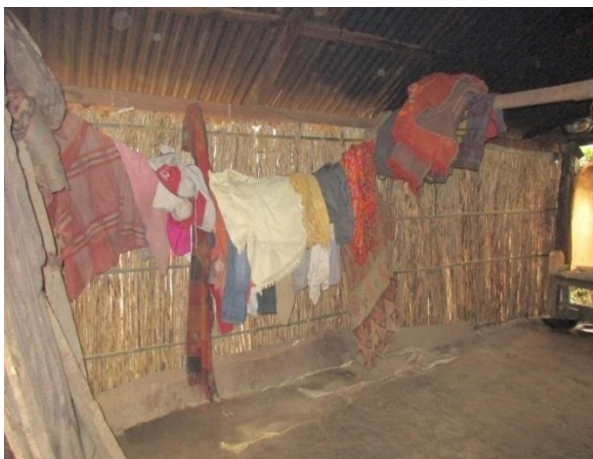
Plate 4.7: Deplorable conditions of Houses, Saraswatipur TG
