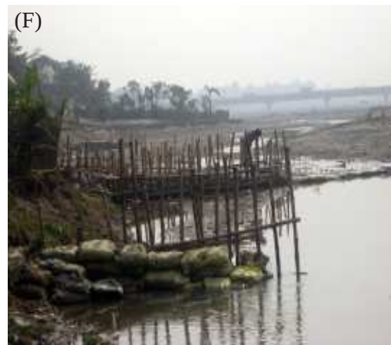
Plate 8.1 Protection of bridge piers from undercutting below Dudhia bridge (A); reconstruction of railway bridge near Matigara (B); protection of embankments (C, D & E); temporarily diversion of channel flows during monsoon period (F).
