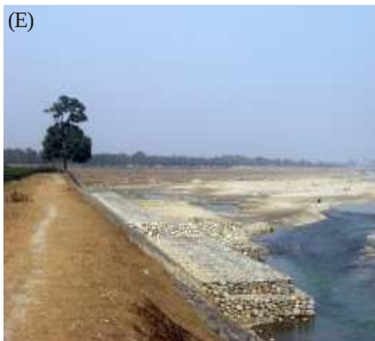
Plate 8.1 Protection of bridge piers from undercutting below Dudhia bridge (A); reconstruction of railway bridge near Matigara (B); protection of embankments (C, D & E); temporarily diversion of channel flows during monsoon period (F).
