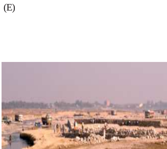
Plate 8.2 Channel flow diversion using sand bags to protect low floodplain settlements (A); construction of boulders filled embankments protection (B, D & E) with plantation of trees (C) and use of sand deposits below embankments for agricultural purposes (F). (Photographs by the Researcher)
