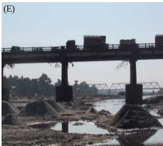
Plate 6.1 The undercutting below Dudhia bridge (A); breached embankment during monsoon flow (B) near Tarabai and railway bridge near Matigara damaged (C) during monsoon high flows; the concentration of channel flow during low flows due to frequent under cutting leaving (D); the undermined Matigara bridge piers (E); and remnants of old flood deposited bars in the lower segment (F) of the lower Balason river. (Photographs by the Researcher)
