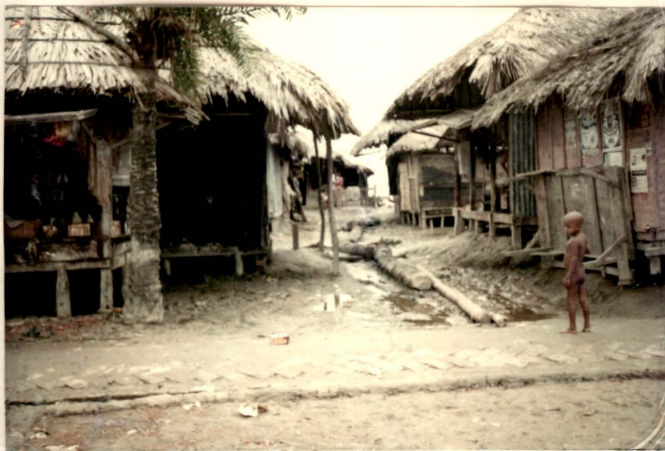
Plate 5.10 Clay road of Rajapur market (inside lane condition)
