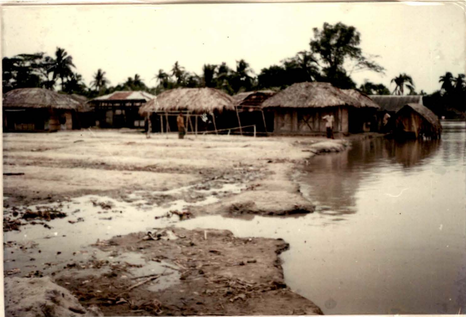
7.7 Dilapidated structure house of market at Khanjahanali.
