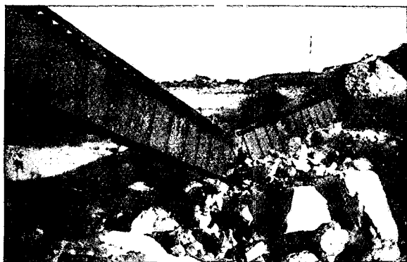
BLOWN-UP BRIDGE AT EPAKO.
