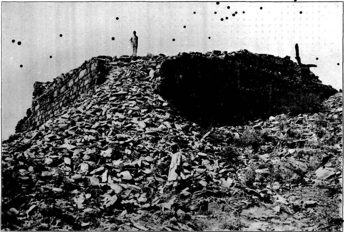
(a) JAMALGARHI: REVETMENT OF CONFERENCE HALL, BEFORE CONSERVATION.
