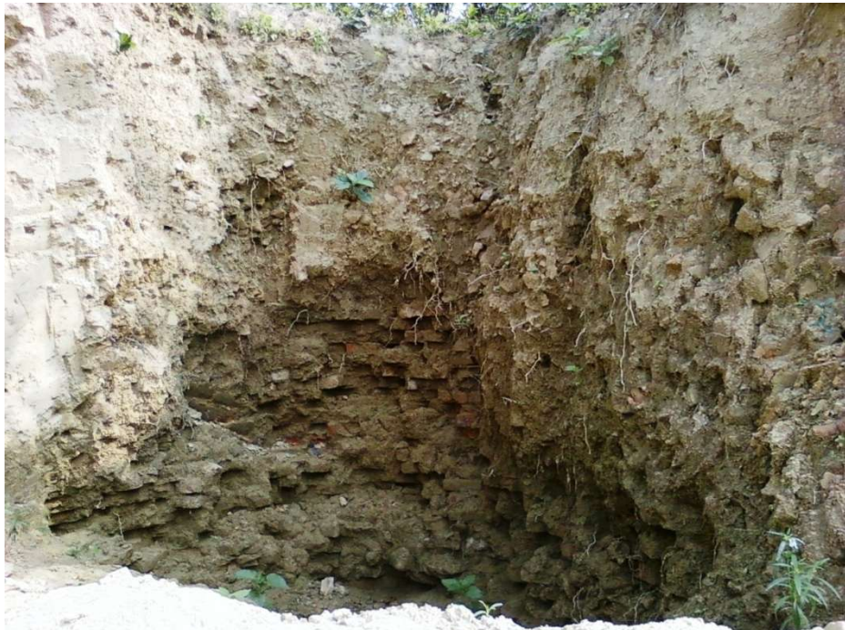
Picture 40: Brick wall of Jagaddala near Mahendra. (photo collected by researcher)
