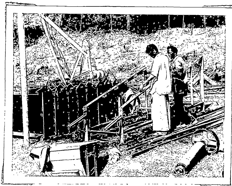
Manufacturing of Tea Machinery (Conveyorbelt) at Bhattacharya Mechanical Engineering Industry Chalsa, Dt. Jalpaiguri.
