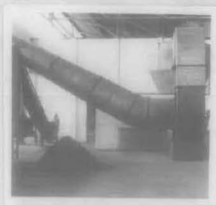
34. The Java Tunnel.
