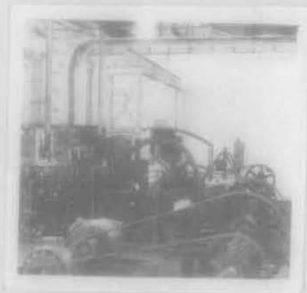
28. The Engine Room.
