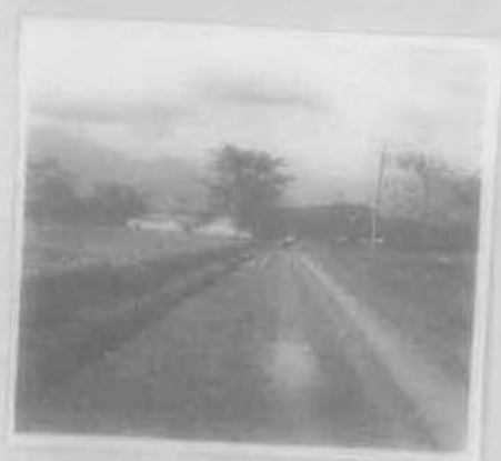
4. Road - planting area on one side.
