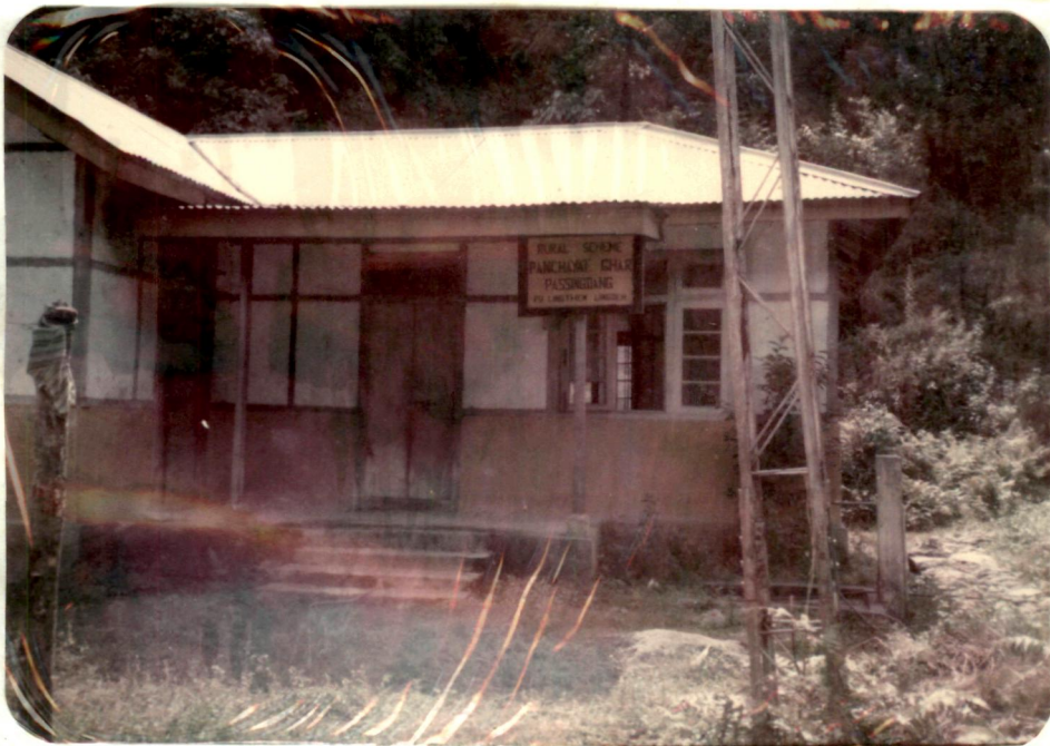
4. PANCHAYAT HOUSE, PASSINGDANG
